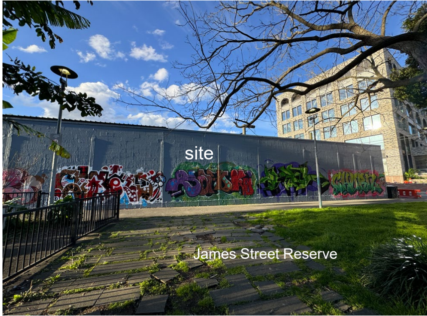
existing southern boundary wall of the site
